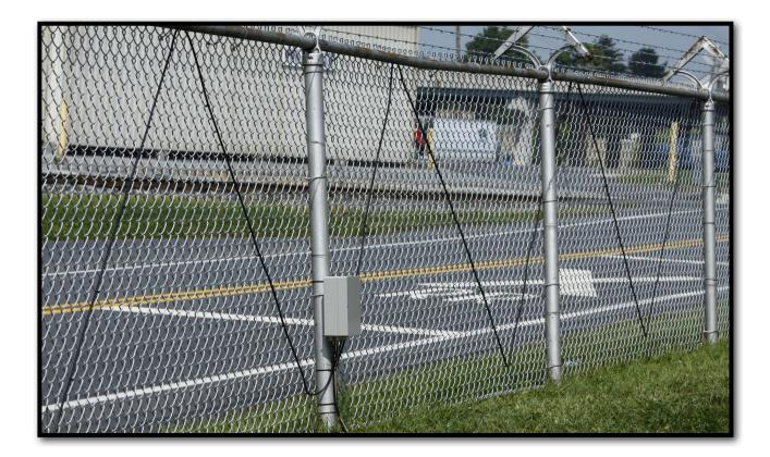
QuadroSense<sup>™</sup> is a special fence protection system. The main part of the system is the control unit, to which vibration sensitive TB cables are connected. The **TB cable** is a special triboelectric cable, which should be attached with cable tie to the fence to be protected, ideally in a sawtoothed or straight line pattern.
